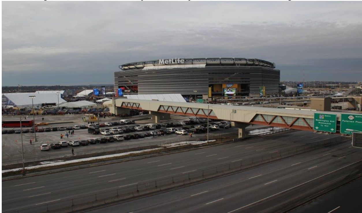
Photo showing Pavilion 6 located behind the pedestrian overpass and Pavilion 5 at the left edge
